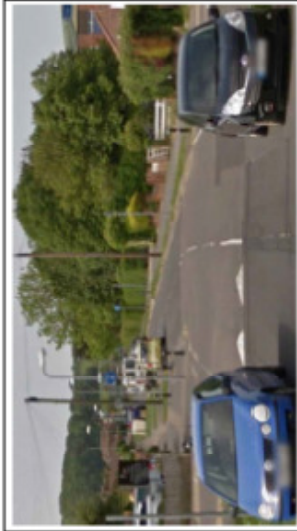
Example of a raised junction. To be used to maintain slower traffic speeds and make it easier for people to cross the road.
