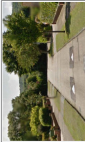
Example of speed cushions. To be used to maintain slower traffic speeds.
