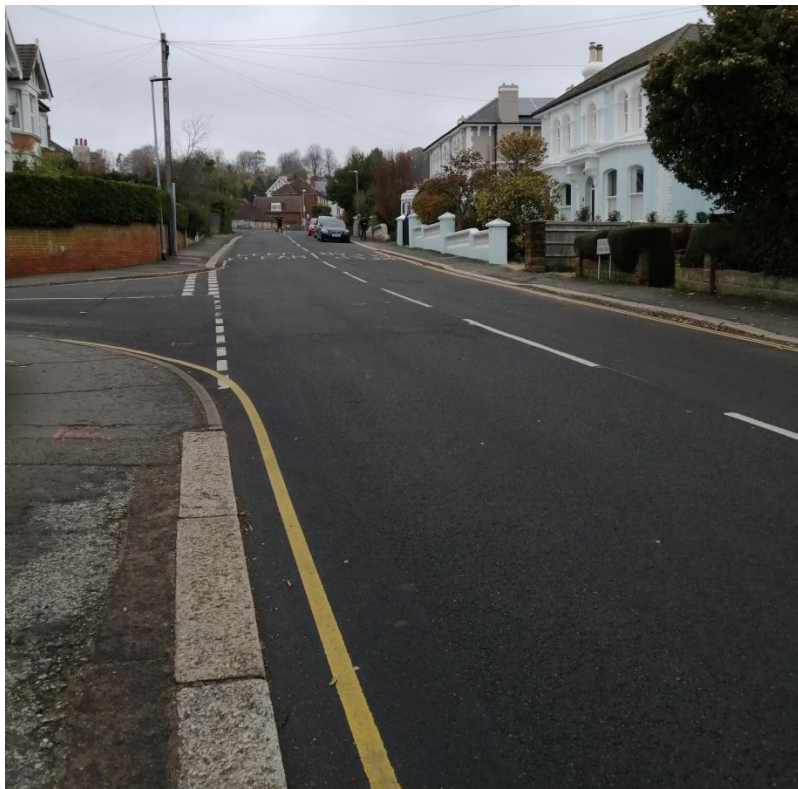
St Helen's Park Road: view northbound towards Freshwater Avenue
