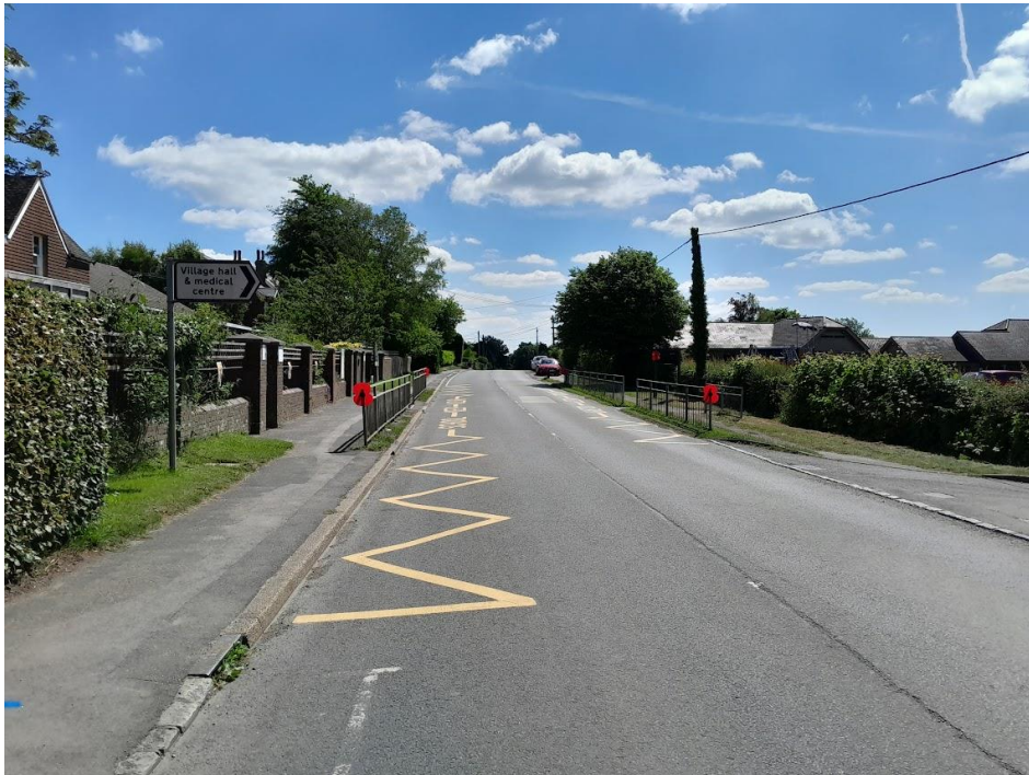
View of 'SCHOOL KEEP CLEAR' yellow zig zag road markings & pedestrian guard-railing outside school entrance for eastbound vehicles on B2096 Battle Road
