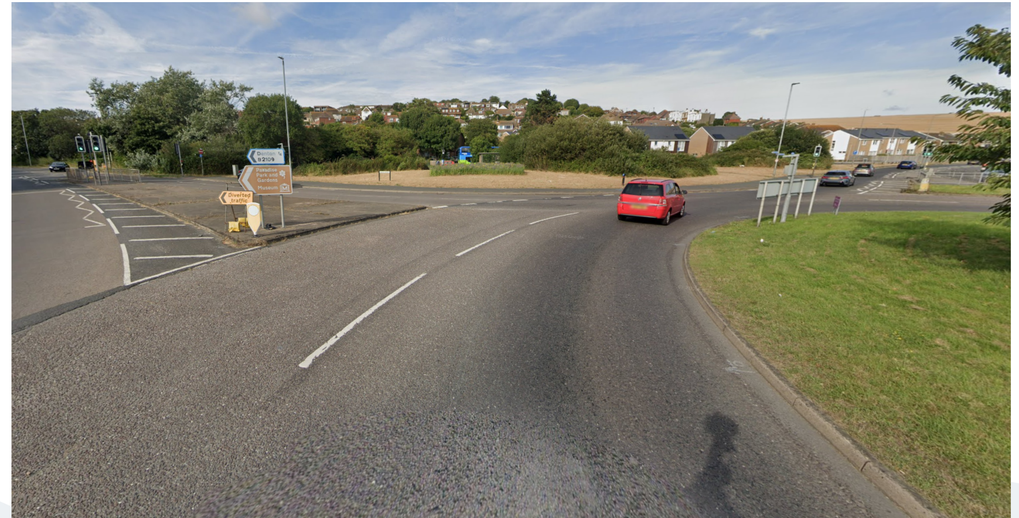
Section of bus lane on the north side of Denton Roundabout.
