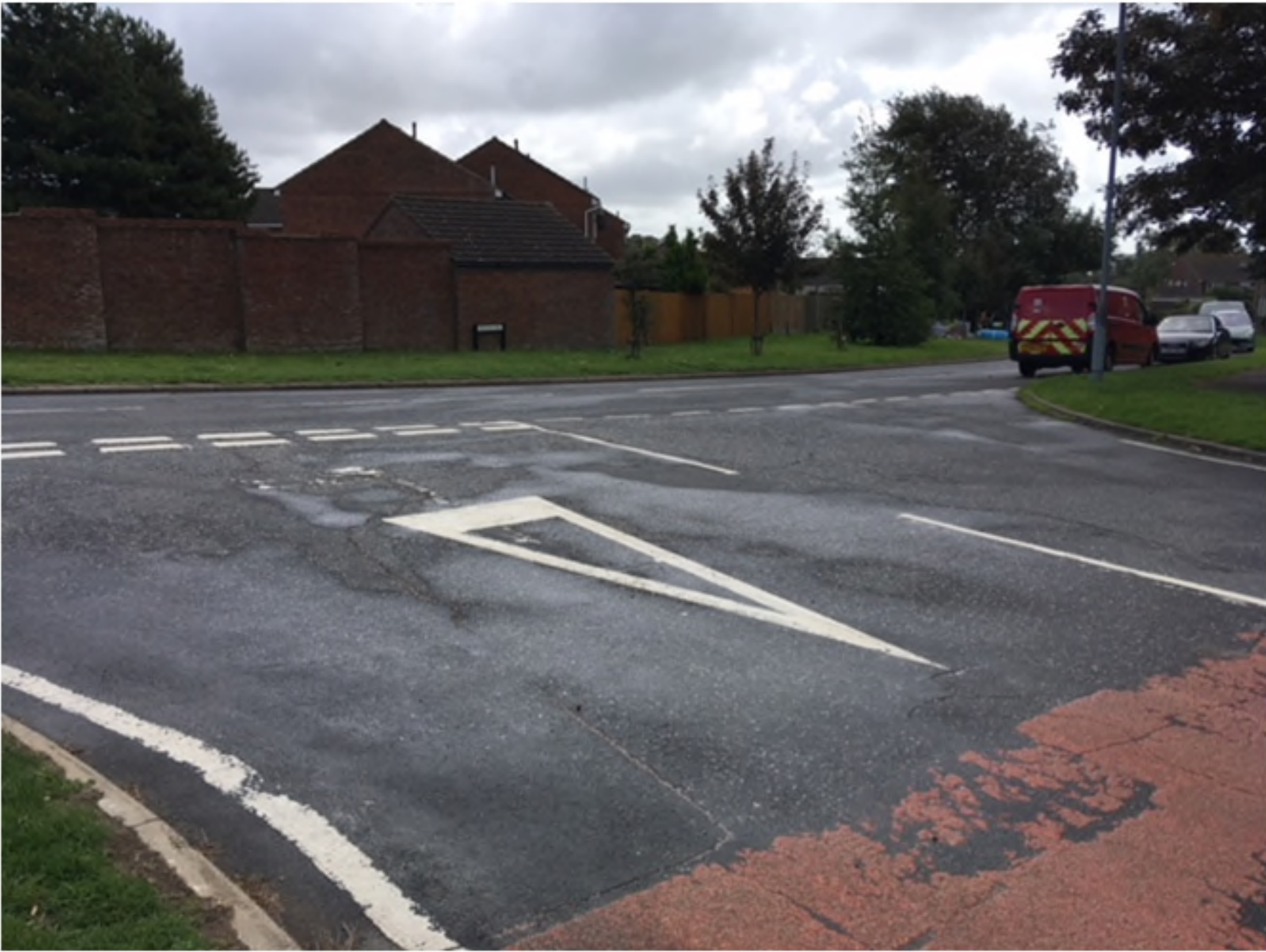
View 1 – Cripps Avenue looking towards its junction with Pelham Rise
