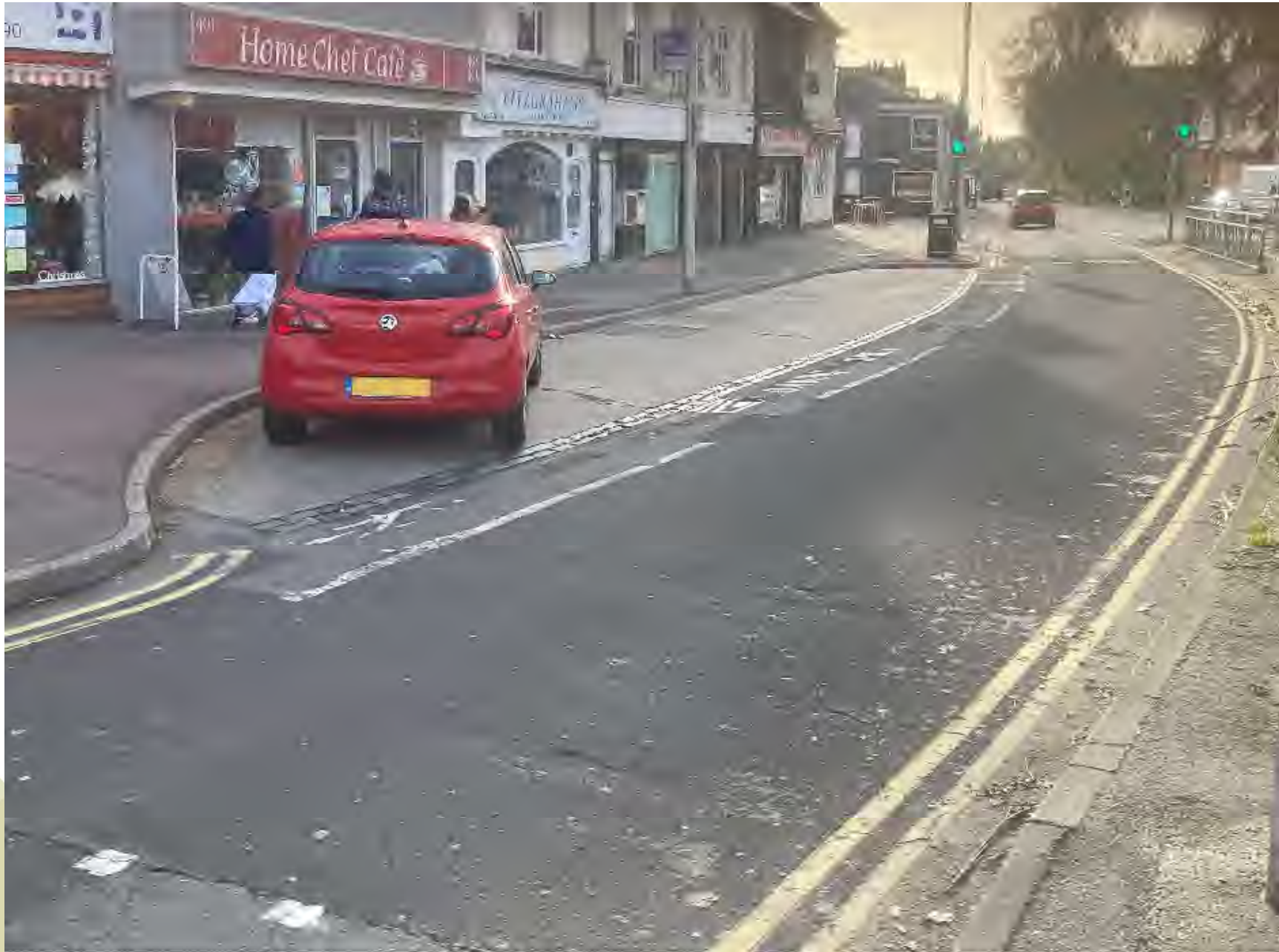
View 1 – Looking south-eastwards at the taxi bay in Sedlescombe Road North
