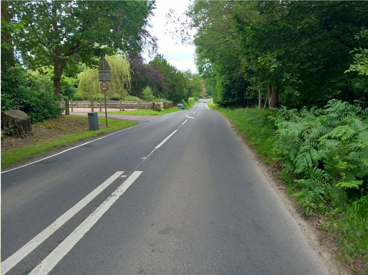
Photo 7 - Geometry and alignment of the A264 on the straighter part of the road without any overtaking restrictions
