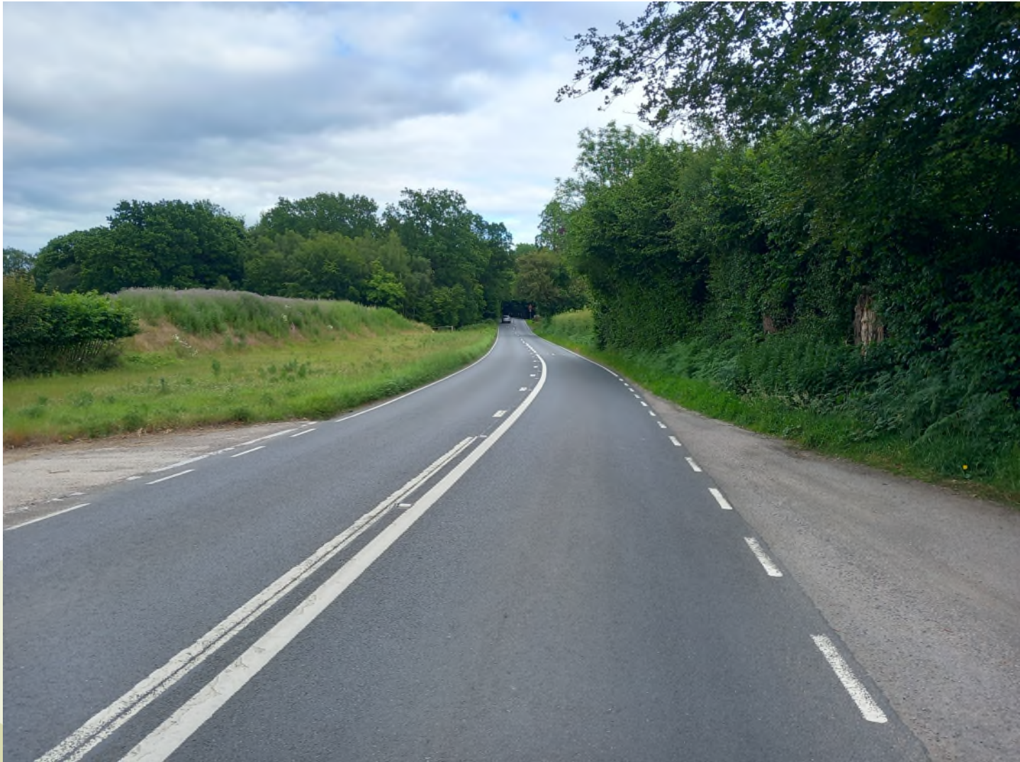
Photo 8 – Geometry and alignment on the A264 on the straighter part of the road with no overtaking restrictions
